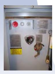
Three position load break switch (Closed-Open-Ground)
