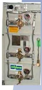
Three Separate 3 Position Switch Closed - Open - Ground
