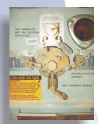
Anti-reverse handle with provision for locks and switch position contacts
