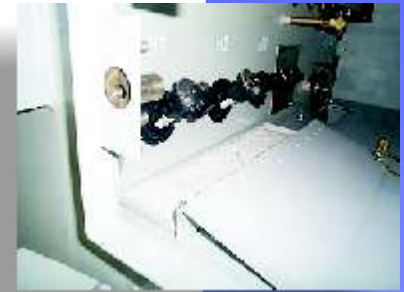
Bay-O-Net fusing and interlock
