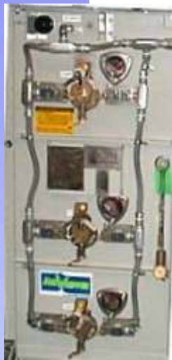
3 Phase loop switch configuration with transformer switch
