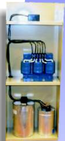
Static Capacitor Bank
