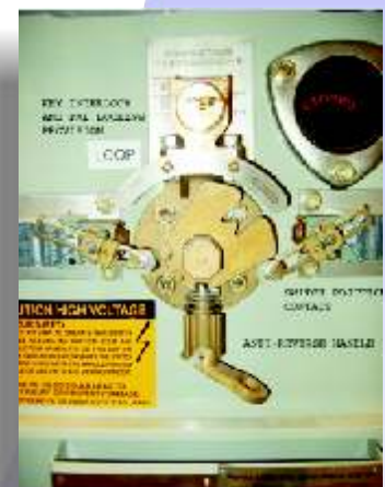
Anti-reverse handle with key locks and switch position contacts
