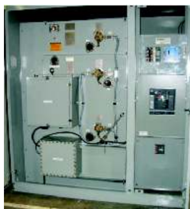
MiniSub with loop switch, vacuum breaker at 27.6 kV, 150 kV BIL, secondary metering, main breaker and TVSS
