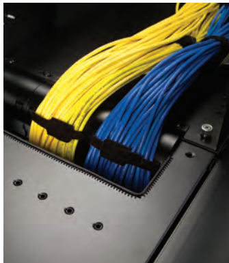
Waterfalls Provide the optimal bend radius for CAT 5e/6 and fiber cables as specified in TIA/EIA-568-A.
