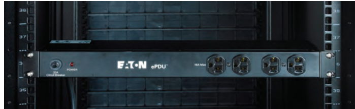
ePDU mounted horizontally in rack
