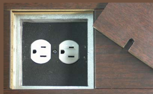
Electrical box cover matches floor finish.
